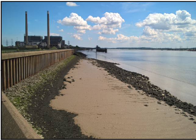
Photograph 1: From left to right: sea wall (wall and rock armour), brown algal beds on intertidal boulders/rocks, and intertidal mudflats.
